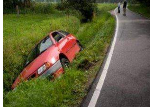
Hazardous Side Ditches
