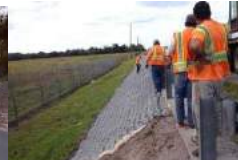
Side Slope Improvements
